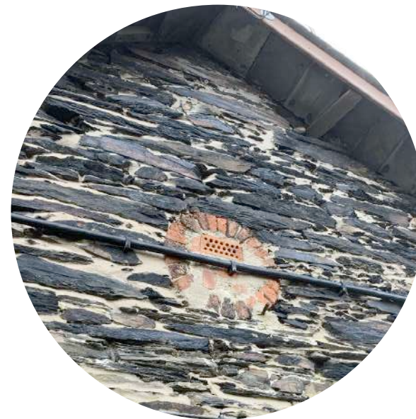
Existing opening is currently blocked and fitted with brick vent - to be reinstated with slate louvre
