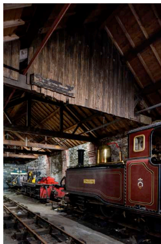
Timber screen detailing - photographs above show vertical boarding with beading (2020)
