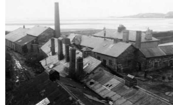
Smithy and foundry in foreground - note the chimneys for each of the hearths, 1956 (John Halsall)
