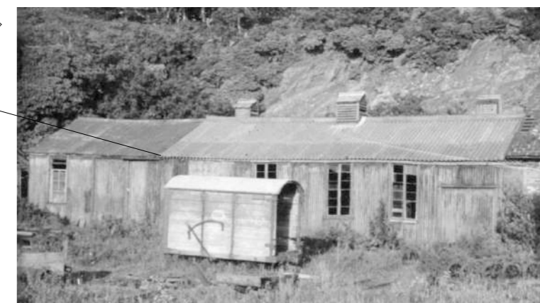
External View of Blacksmiths Extension
