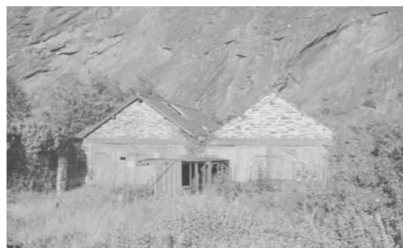
Old Carriage Shed - extension on the right before demolition, 1958 (David Ronald)
